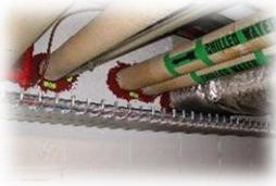
Contractors installing cables, pipes in buildings are obliged to fire stop cable holes through which they have cabled as part of the contract. All cable holes through floors and compartment walls must be fire stopped to prevent passage of fire, smoke and hot gases.
